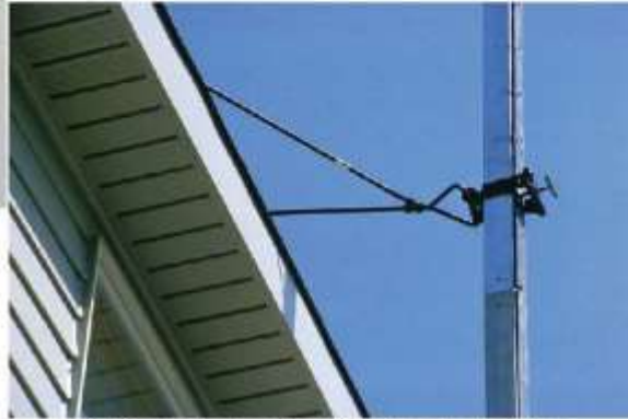
A Pump Jack scaffold's triangular bracing.
