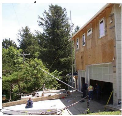
guided the pole with a rope. One of the workers on the ground secured the pole's rubber base plate while the other worker walked the pole up to a vertical position about three feet from the front of the garage.
